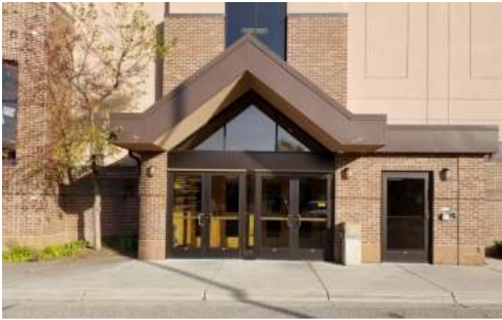
Park Avenue Methodist
